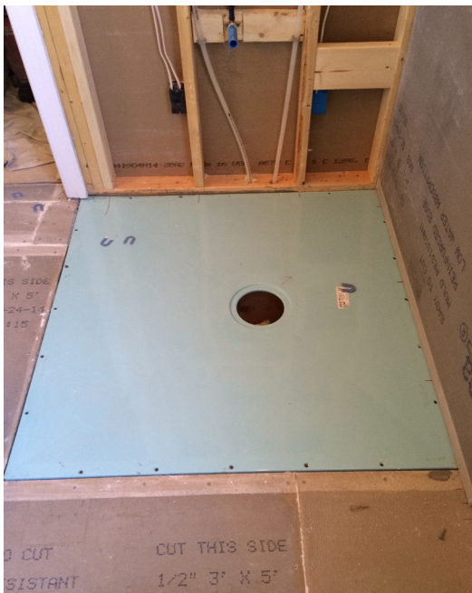
Classic shower base installed on joists.
